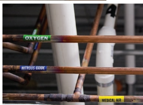
The full basement houses the mechanical equipment and provides full access to wiring, piping and plumbing for each operator.
